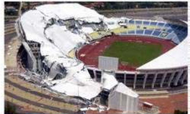
Both contractors responsible for the construction and the clearing of debris at the Sultan Mizan Stadium in Kuala Terengganu were said to be "unregistered and inexperienced." (Photo credit: sokernet.com)
