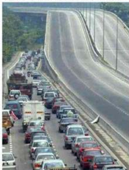
The Government has yet to reveal the outcome of the investigation into the defective flyover between the Taman Bukit Maluri and FRIM interchange worth RM238 million (Photo credit: elections.thestar.com.my)
