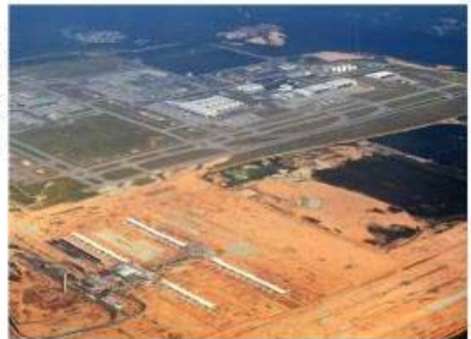
KLIA 2 under construction ( http://www.klia2.info/photos/work-in-progress )
